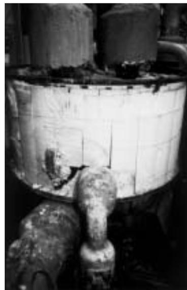
19a Asbestos-insulated vessel and supply pipes in a factory.
