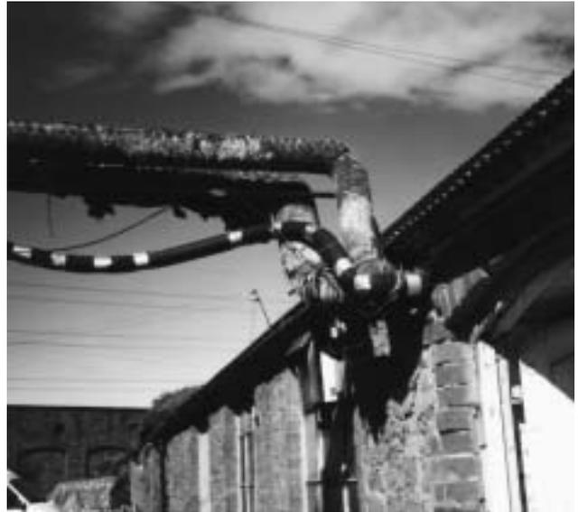
3h Badly degraded external asbestos-lagged pipe in an industrial plant, with asbestos rope wound around the bends.
