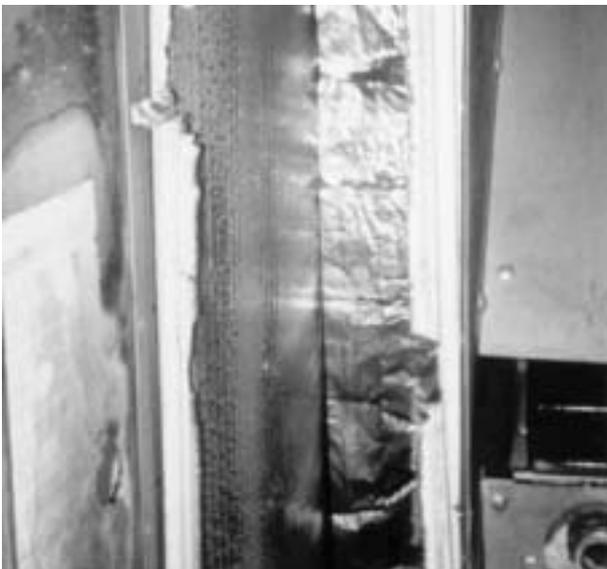
7b Foil-backed asbestos cardboard insulation inside a warm air heater.
