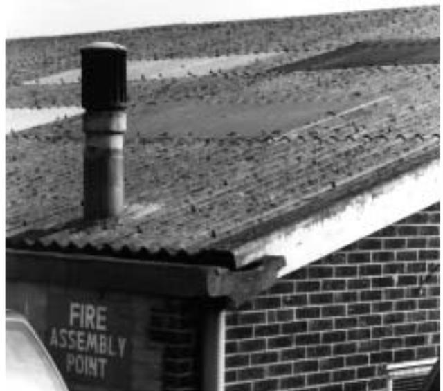
11c Asbestos cement external flue, rain water gutter and profile roofing sheet.
