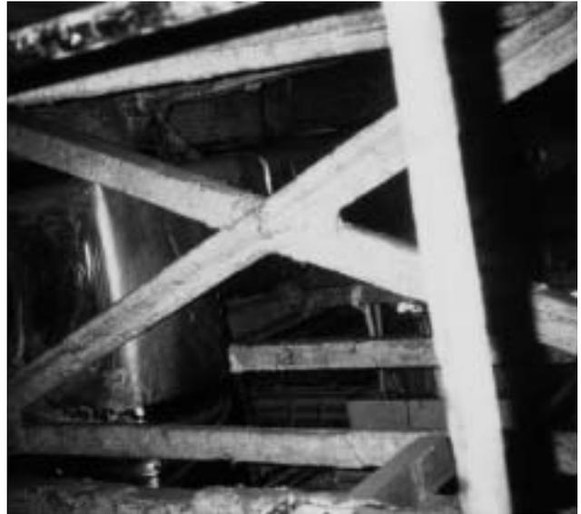
2c Sprayed amosite fireproofing on steel roof support beams in a return air plenum showing signs of damage and wear at the bottom caused by access for maintenance.
