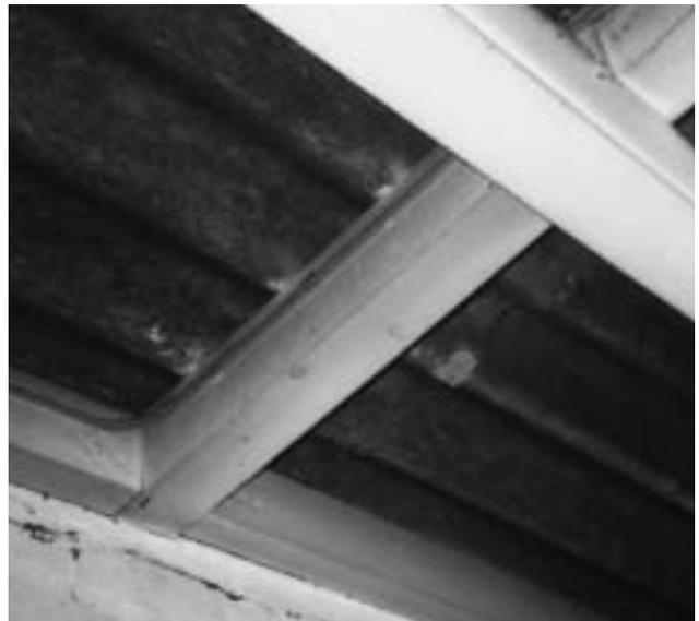
10a Asbestos cement roof (seen from inside).
