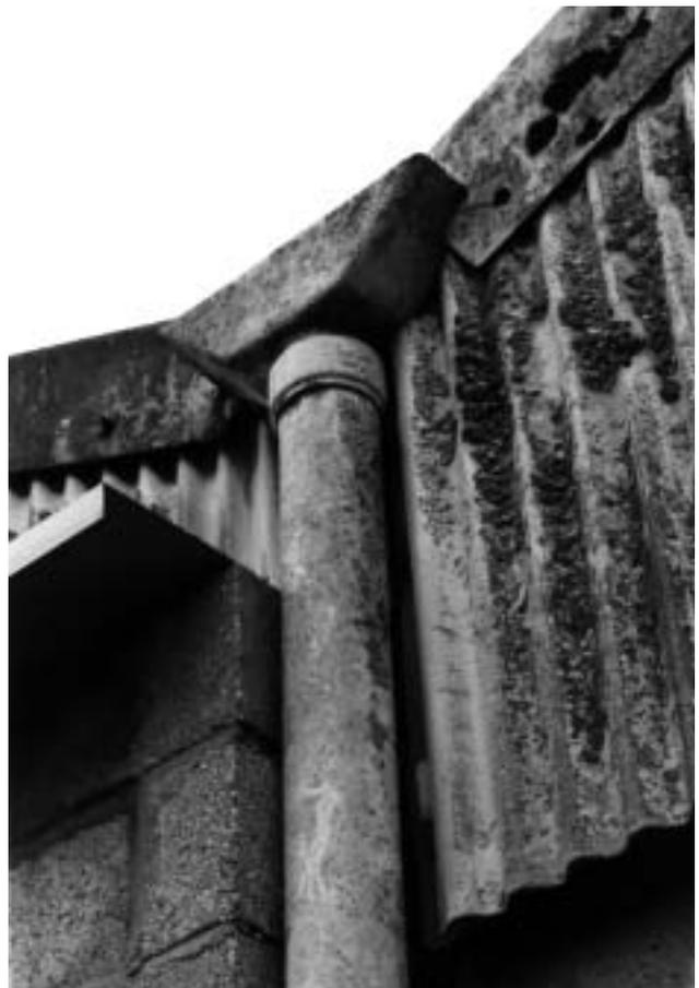
11d Asbestos cement downpipe, hopper and profile sheet.
