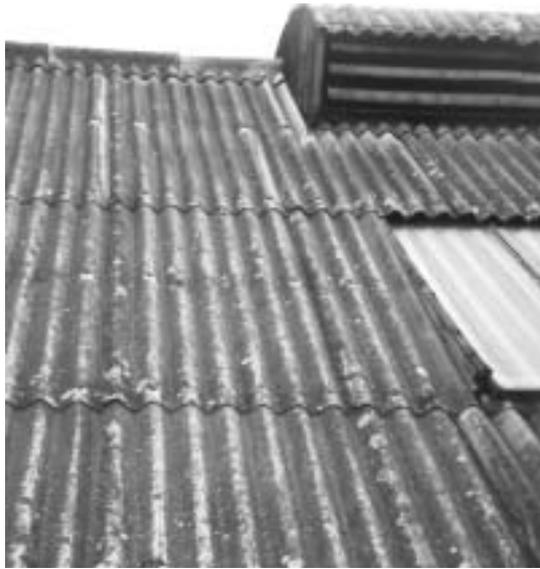
10b Asbestos cement roof (weathered exterior).
