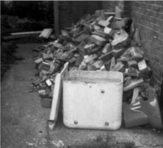
11a Asbestos cement water tank.
