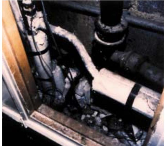
20a Asbestos debris in the bottom of a service riser.
