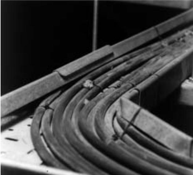
20c Fibrous debris in a cable tray.
