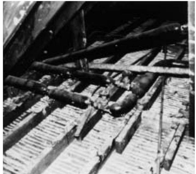
3a Asbestos-insulated water pipes in a loft, sealed and in good condition.
