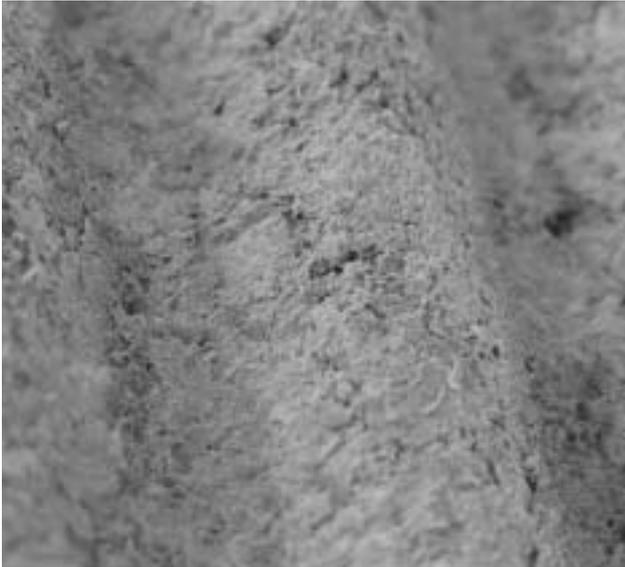
2e Close-up of the surface of sprayed amosite insulation (~40 mm thick) on the underside of an asbestos cement roof.
