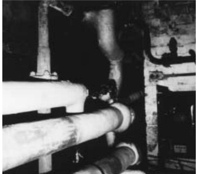
*3d Asbestos pipe lagging on central heating pipes at the entrance of an underground crawl tunnel to adjacent premises.*
