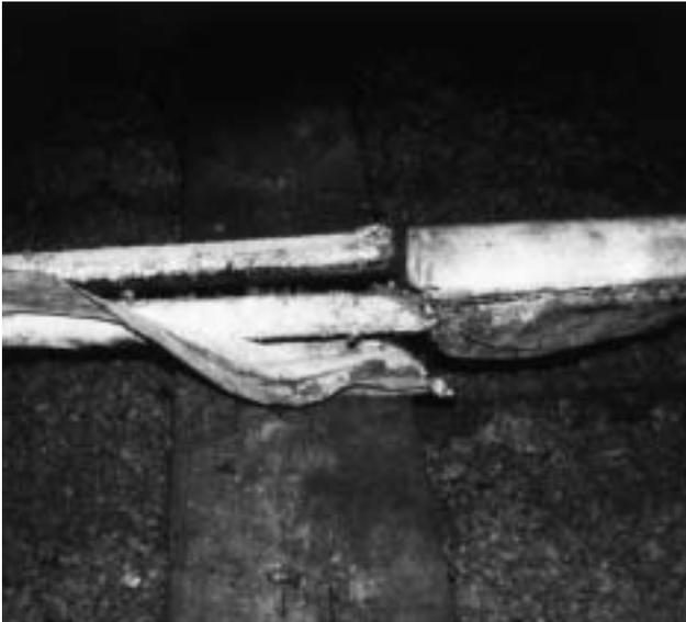
*3b Asbestos-insulated water pipes in a loft, showing evidence of maintenance work damage, with detached pre-formed sections and calico wrapping.*
