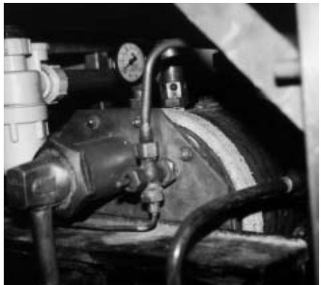
8a Example of asbestos tape on a domestic water heater.
