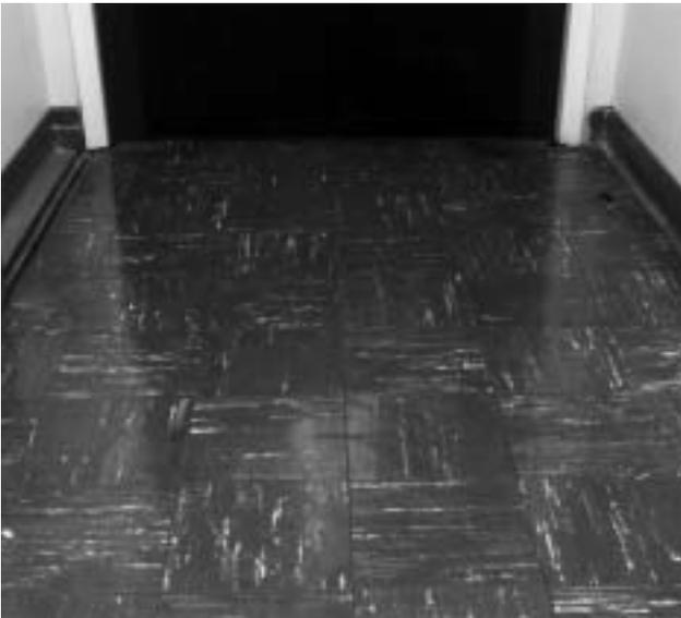
14a Asbestos-containing vinyl floor tiles.
