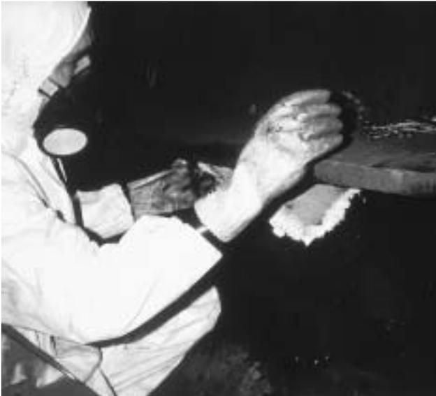
4a Removal of a piece of low density millboard from an electrical cable box.
