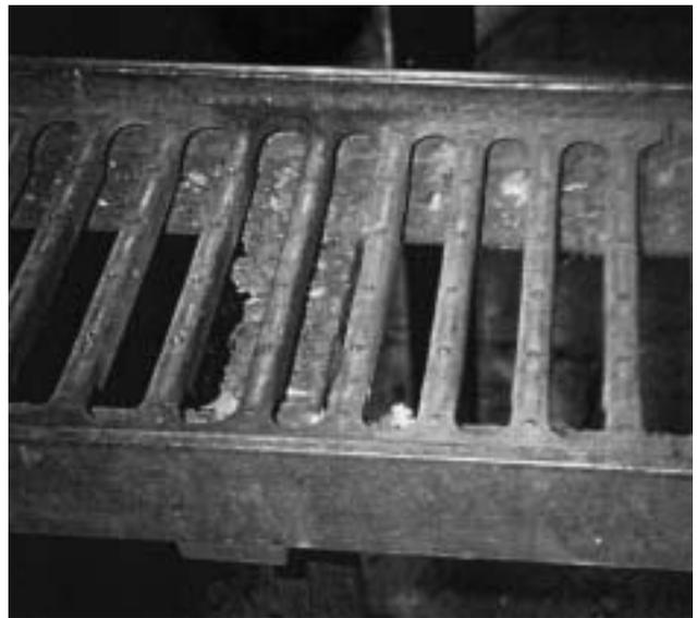
20b Asbestos debris left on a walkway.
