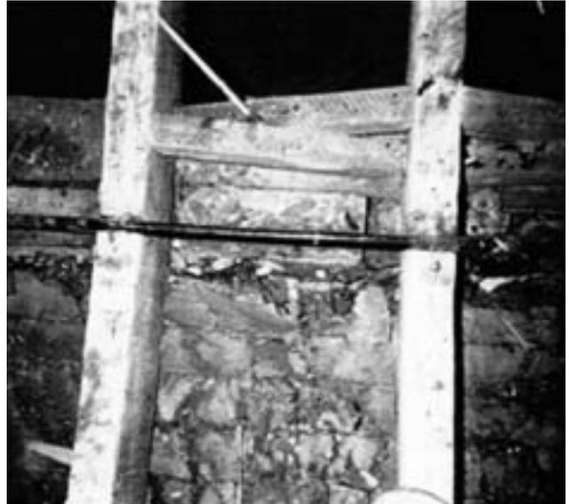
1b Loose insulation with paper cover degraded under a dance floor.
