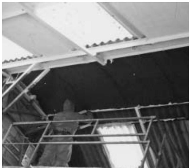
2d Sprayed crocidolite asbestos (100 mm thick) applied as thermal insulation to the underside of an asbestos cement roof. From top to bottom, the encapsulated spray, the spray without encapsulant and removed spray from the A/C cement sheets.
