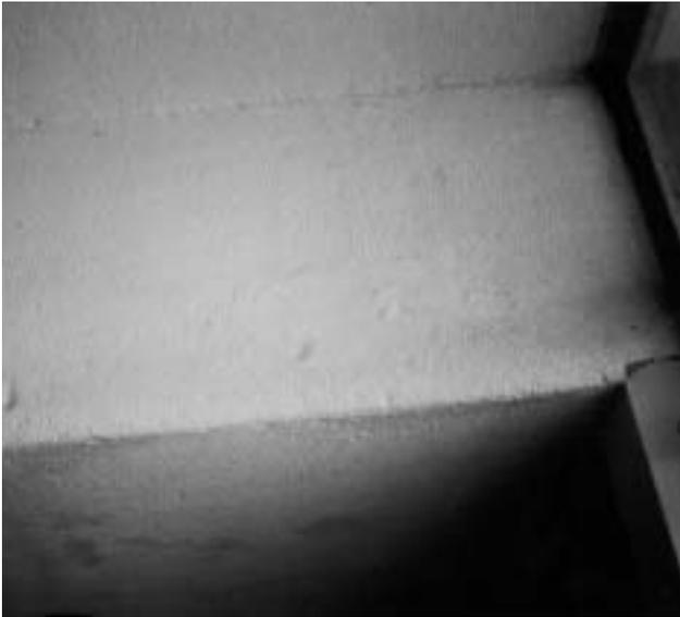
2a Cementitious sprayed chrysotile asbestos on a ceiling for decorative and fireproofing purposes, showing evidence of previous damage and repair.
