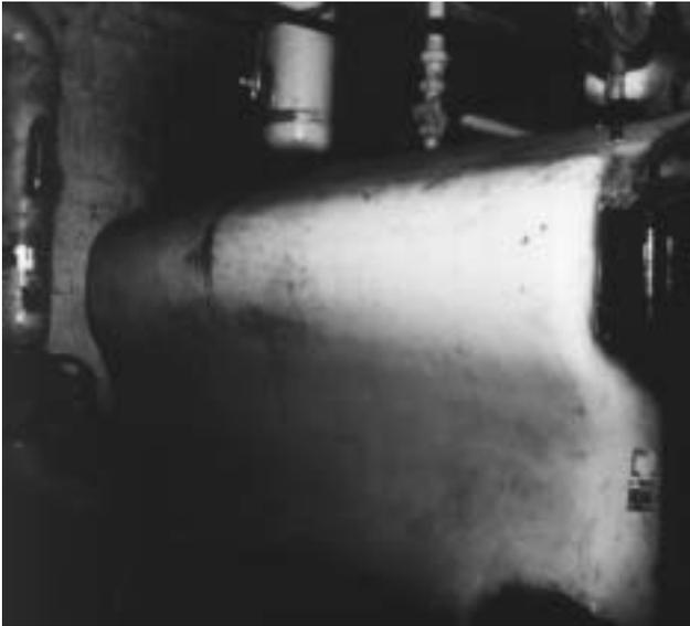
3f Asbestos-lagged boiler with a hard plaster coating.
