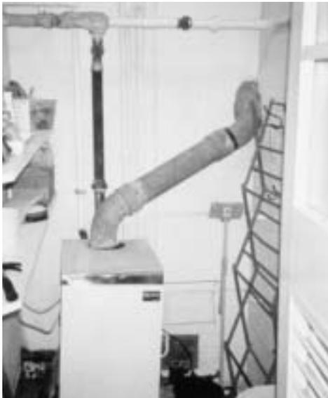
11b Asbestos cement flue from a domestic boiler.
