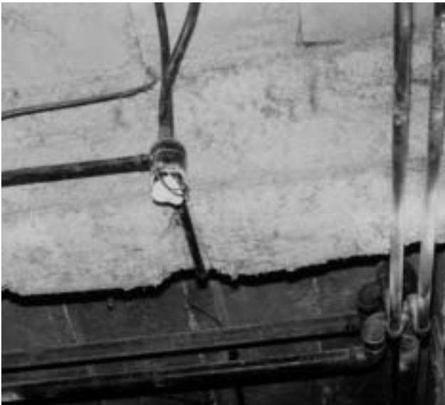
2b Poorly tamped sprayed chrysotile fireproofing on a structural steel beam holding up a concrete floor showing some overspray onto the concrete and damage by electrical work.
