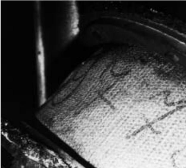
8b Asbestos gaiter between pipe flanges.
