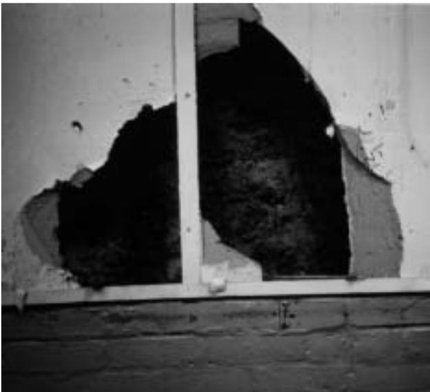
2f Sprayed crocidolite thermal insulation applied to external wall cladding and enclosed behind non-asbestos wallboard.
