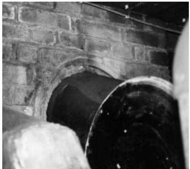
8e Asbestos rope used as packing/seal where pipe passes through a wall.
