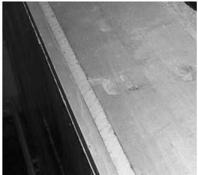
6a AIB inside an interior wall faced with plasterboard.
