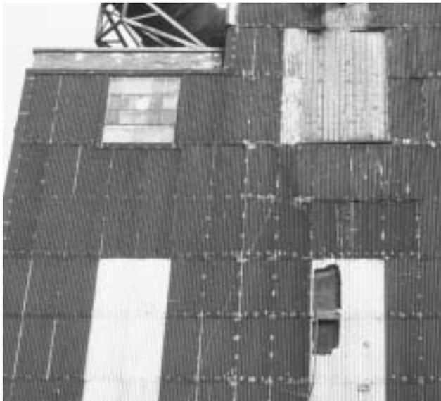
10c Asbestos cement vertical cladding.
