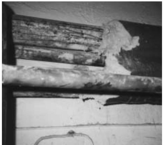
3i Example of hand-applied 'hard set' insulation, partially removed from a pipe.
