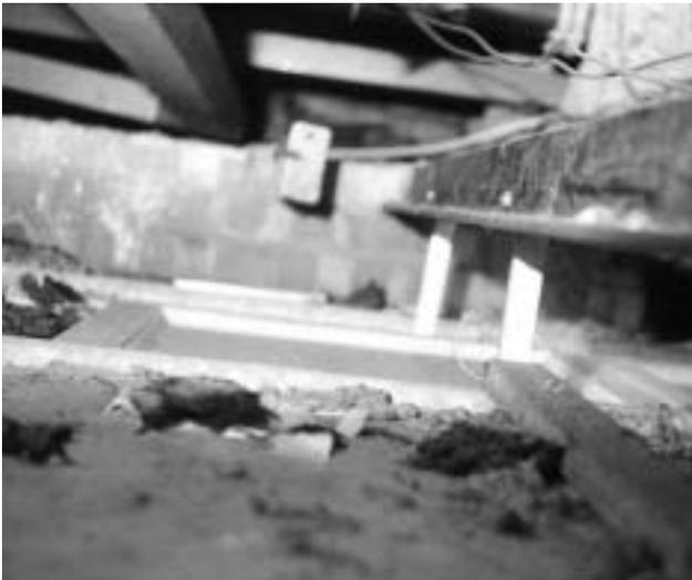
20d Sprayed asbestos debris released onto a suspended ceiling from cable installation work.
