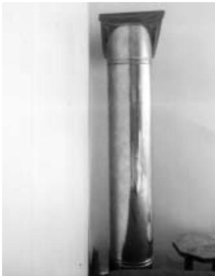
16a Metal-clad asbestos flue pipe.
