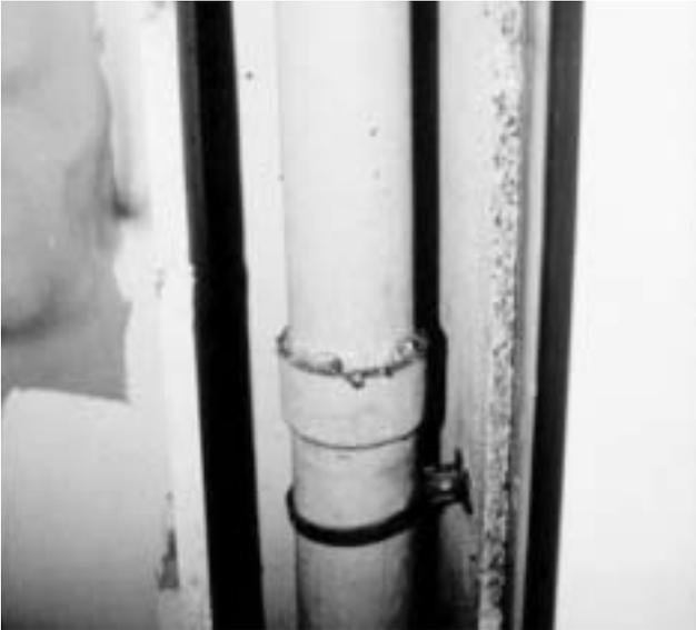
5d AIB around a service riser shaft (showing cut and uncut edges).
