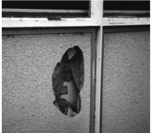
5a Typical use of AIB in system-built flats. The internal AIB panel is visible behind a broken flat sheet (possibly asbestos cement) with textured coating (possibly chrysotile asbestos-containing) with MMMF insulation in between.
