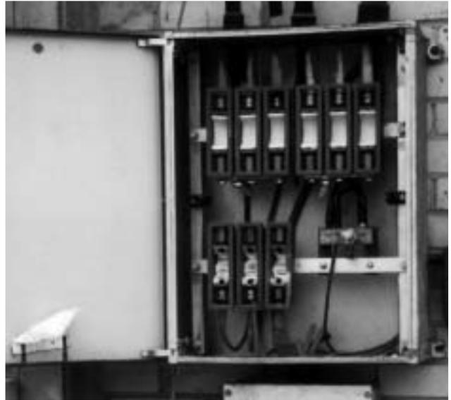
18c Asbestos tape flash guards in a fuse box.
